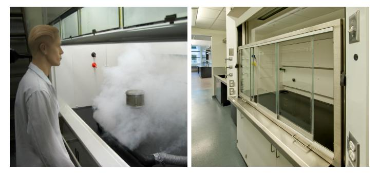
Laboratory fume hoods are safety devices where hazardous chemicals can be handled safely while the fumes and vapors they generate are exhausted out of the building through a specialized ventilation system. Regular, periodic testing of laboratory fume hoods is critical to maintaining effective operation and ensuring the health and safety of your research staff.
